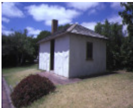
mccrae homestead charles street mccrae kitchen rebuilt
