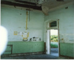
B5431 Railway Station, Koroit pre restoration
