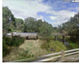
B6521 GoogleEarth Image Ellerslie Bridge
