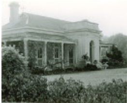
B2845 Kirkella Homestead, Campbells Bridge
