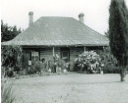
B1837 Chock & Log Cottage, Poowong
