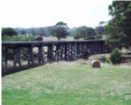
B6952 Tarwin River East Branch Railway Bridge
