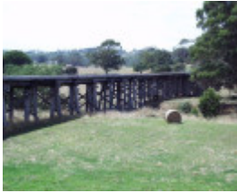
B6952 Tarwin River East Branch Railway Bridge
