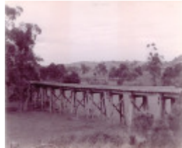
B6952 Tarwin River East Branch Railway Bridge
