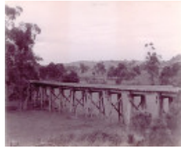
B6952 Tarwin River East Branch Railway Bridge
