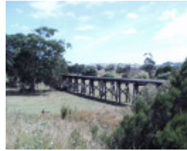
B6952 Tarwin River East Branch Railway Bridge
