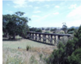
B6952 Tarwin River East Branch Railway Bridge
