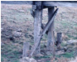
B6909 Railway Bridge
