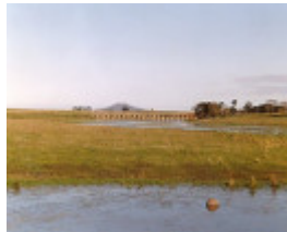
B6909 Railway Bridge
