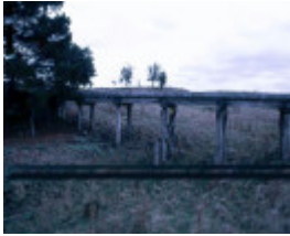
B6909 Railway Bridge
