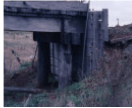
B6909 Railway Bridge
