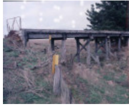
B6909 Railway Bridge
