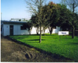
B6936 Hamilton Gasworks
