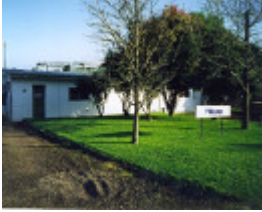
B6936 Hamilton Gasworks
