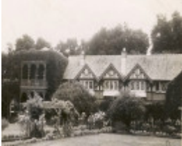
B0062 Murndal Homestead Murndal Rd Hamilton
