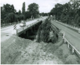
B1743 Hughes Bridge Hume Hwy Avenel
