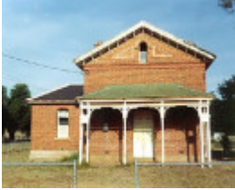
B1538 Fmr Court House Queen St Avenel
