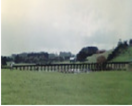
B6911 Rail Bridge Dennington
