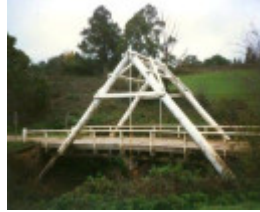
B6838 Hiawatha A Frame Bridge
