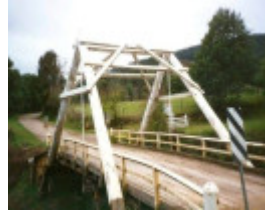
B6838 Hiawatha A Frame Bridge
