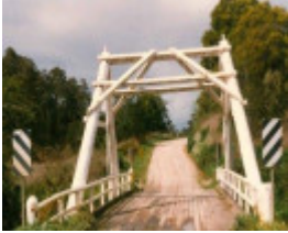
B6838 Hiawatha A Frame Bridge
