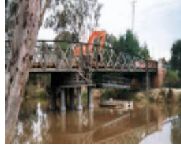
B2379 Swing Bridge Being Renovated
