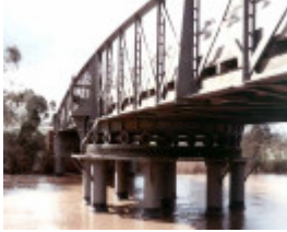
B2379 Swing Bridge
