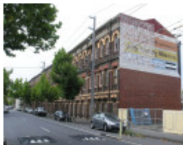
FORMER DENTON HAT MILLS SOHE 2008
