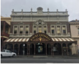
Former Mining Exchange
