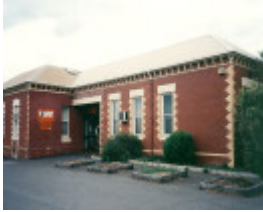
B6512 Wodonga Railway Station Complex
