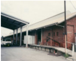
B6512 Wodonga Railway Station Complex
