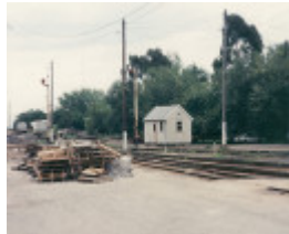
B6512 Wodonga Railway Station Complex
