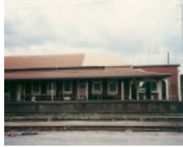
B6512 Wodonga Railway Station Complex
