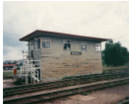
B6512 Wodonga Railway Station Complex
