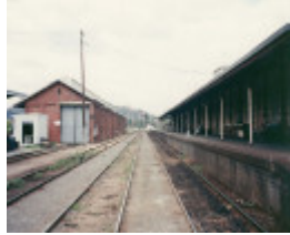
B6512 Wodonga Railway Station Complex
