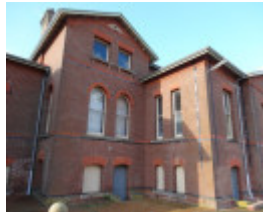
B2371 Serviceton Station street front
