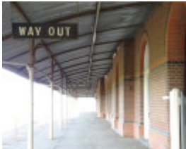
B2371 Serviceton Station verandah
