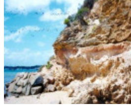
L10051 Erosion on Coastline
