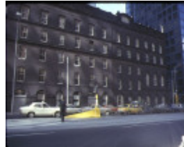
1 goldsbrough mort building bourke rd melb view front
