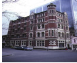
1 former gollin & amp; company building bourke street melbourne frnt view
