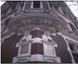
former gollin & company building bourke street melbourne front detail
