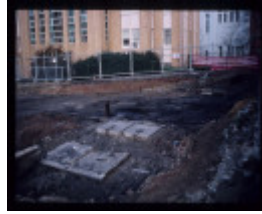
CAMP STREET PRECINCT EXCAVATION
