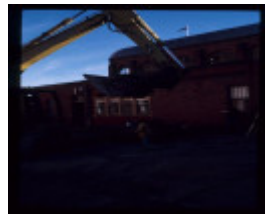
CAMP STREET PRECINCT EXCAVATION
