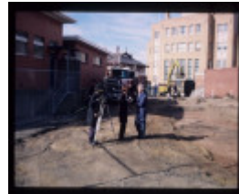
CAMP STREET PRECINCT EXCAVATION
