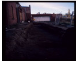
CAMP STREET PRECINCT EXCAVATION
