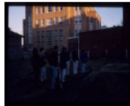
CAMP STREET PRECINCT EXCAVATION
