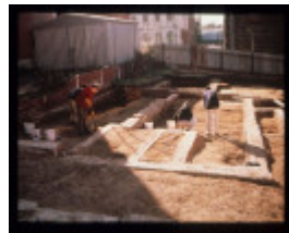
CAMP STREET PRECINCT EXCAVATION
