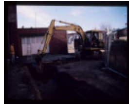
CAMP STREET PRECINCT EXCAVATION
