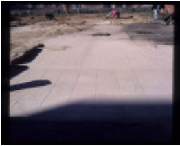
CAMP STREET PRECINCT EXCAVATION
