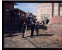
CAMP STREET PRECINCT EXCAVATION
