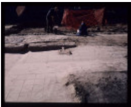
CAMP STREET PRECINCT EXCAVATION
