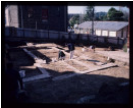
CAMP STREET PRECINCT EXCAVATION
