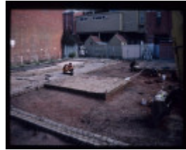
CAMP STREET PRECINCT EXCAVATION
