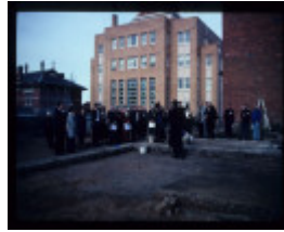
CAMP STREET PRECINCT EXCAVATION
