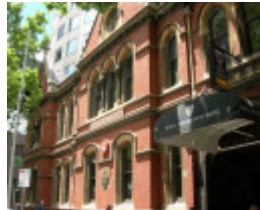
OLD BOURKE STREET WEST POLICE STATION AND CELL BLOCK SOHE 2008
