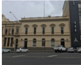
Former Bank of NSW
