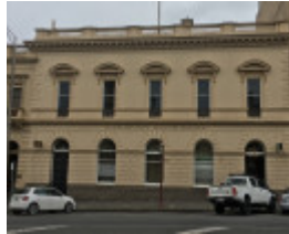
Former Bank of NSW 2
