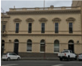
Former Bank of NSW 3
