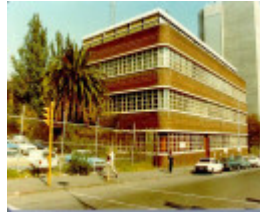
1 rmit building no 9 rear view 1982
