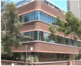
RMIT BUILDING NO. 9 SOHE 2008
