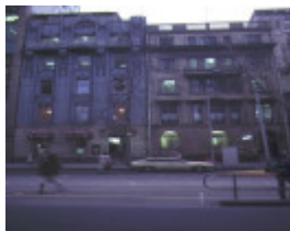
1 victor horsley chambers collins street melbourne front view
