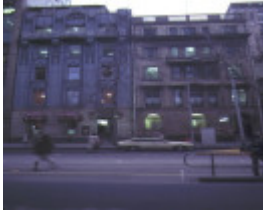
1 victor horsley chambers collins street melbourne front view
