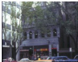
1 melville house collins street melbourne front view
