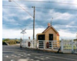
B7315 New St Railway Gates
