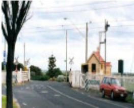
B7315 New St Railway Gates
