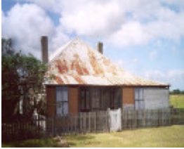
B7316 Former Commercial Hotel
