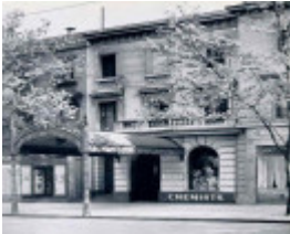
ogg & company demolished 76 collins street front view
