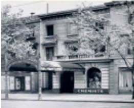
ogg & company demolished 76 collins street front view
