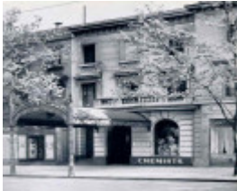
ogg & company demolished 76 collins street front view
