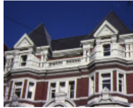
austral building collins street melbourne detail external top floor
