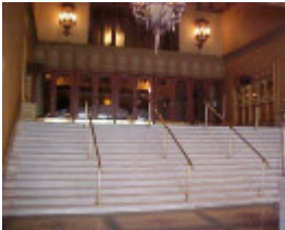
regent theatre collins street entrance steps jul1999
