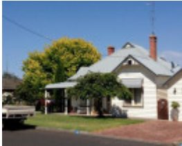
House, 42 Brown St
