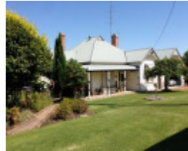
House, 42 Brown St
