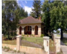
Former UV Knight's House, 26 Ogilvy St
