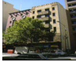
1 newspaper house collins street melbourne front view feb1986
