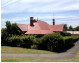
House, 19 Long St
