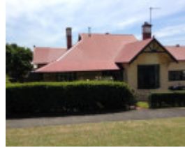
House, 19 Long St
