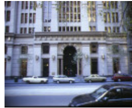
banking chamber commercial bank of australia external entrance
