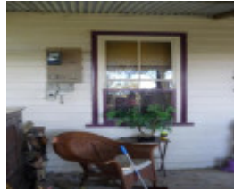
Window detail, House, 1790 Grand Ridge Rd
