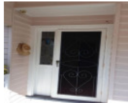
House, 21 Bridge Street
