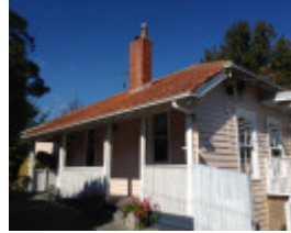
House, 21 Bridge Street
