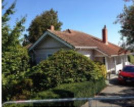
House, 21 Bridge Street
