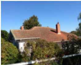
House, 21 Bridge Street
