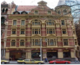
1 winfield building collins street melbourne front view sep1999
