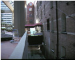
rialto building melb taberet- entrance
