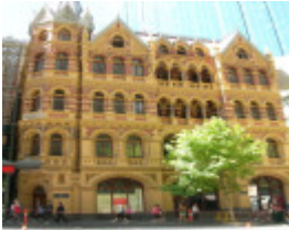
RIALTO BUILDING SOHE 2008
