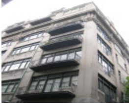
DOVERS BUILDING SOHE 2008
