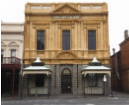
BALLARAT ART GALLERY_Restored Facade_Compressed.jpg 2010
