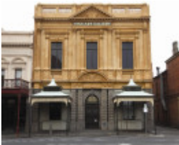
BALLARAT ART GALLERY_Restored Facade_Compressed.jpg 2010
