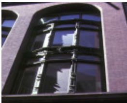
royston house flinders lane melbourne detail of front window feb1980
