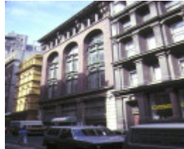
1 royston house flinders lane melbourne front view mar1985
