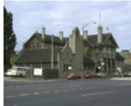
missions to seamen flinders street extension melb side elevation feb1986
