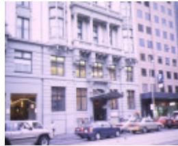
commercial travellers association building flinders street melbourne front entrance view sep1998
