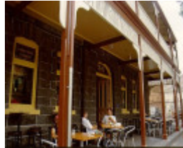
macs hotel franklin street verandah january 2000
