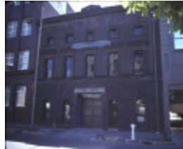
former zanders no3 warehouse king street melb front view
