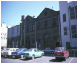
former levicks & piper wholesale ironmonger's warehouse king street melb rear view
