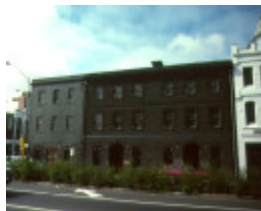
1 h66 former f blight king street
